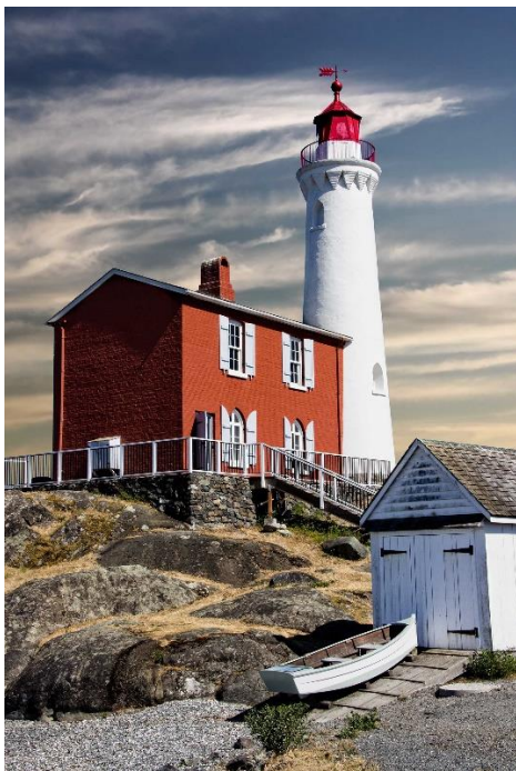
Fisgard, National Historic Site of Canada. Colwood, British Columbia.
